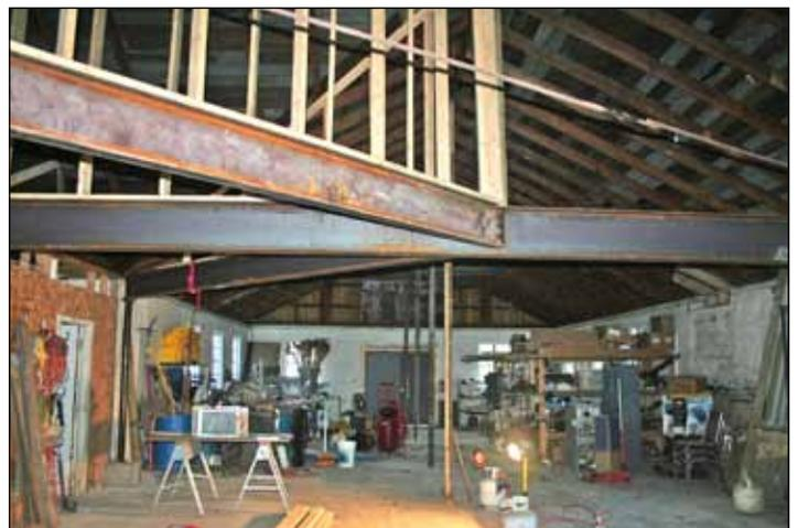
**Fixed Shop roof that was failing - addition of three steel beams**
