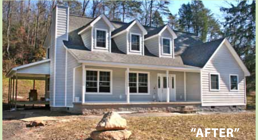
Nearly completed residence for Yankey family as of November 20, 2012
